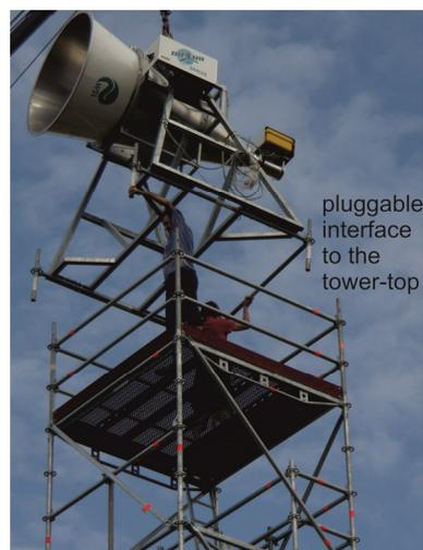
**Figure 2:** Installation of ELBARA on the tower at the Valencia Anchor Station (VAS). A mechanical interface (vertical tubes) pluggable to the tower structure (vertical rods) was attached to the bottom of the scaffold to facilitate the installation with the aid of a crane.
